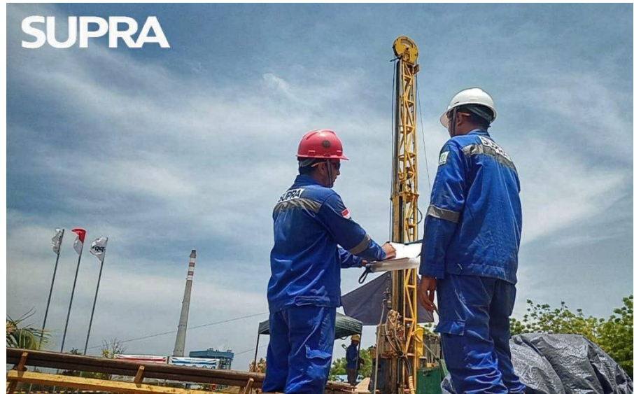
Figure : SUPRA's professional drilling analyzing cost benefit of the well construction
